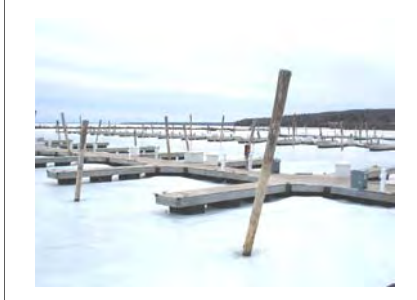
Port Superior Marina pelican posts and piers in the winter “jack out” from ice movement.
